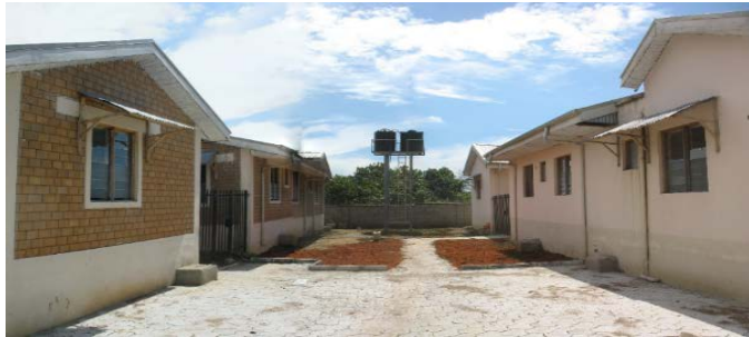
PLATE 3.1 RESIDENTIAL BUILDING IN NIGERIA SHOWING ROOF EAVES AND AWNINGS
